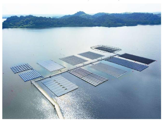
The team also assessed other potential deployment options, such as Floating Solar on reservoirs and near-shore. Image shows the 1  $MW_p$  Floating PV testbed on Tengeh Reservoir in Singapore. (Photo: SERIS)
